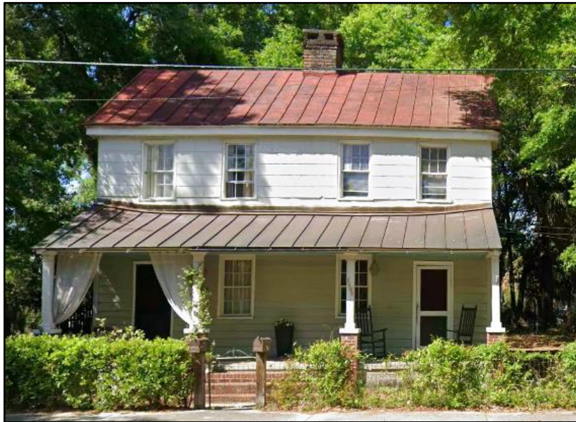
C. 1103 Greene Street: Picture of historic duplex (Google Maps, Apr. 2026)
