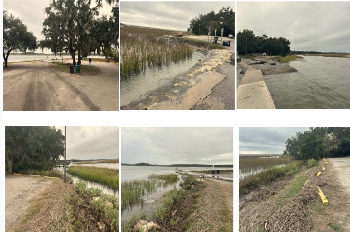
PIGEON POINT LANDING - EXISTING CONDITIONS AND AREAS OF CONCERN
