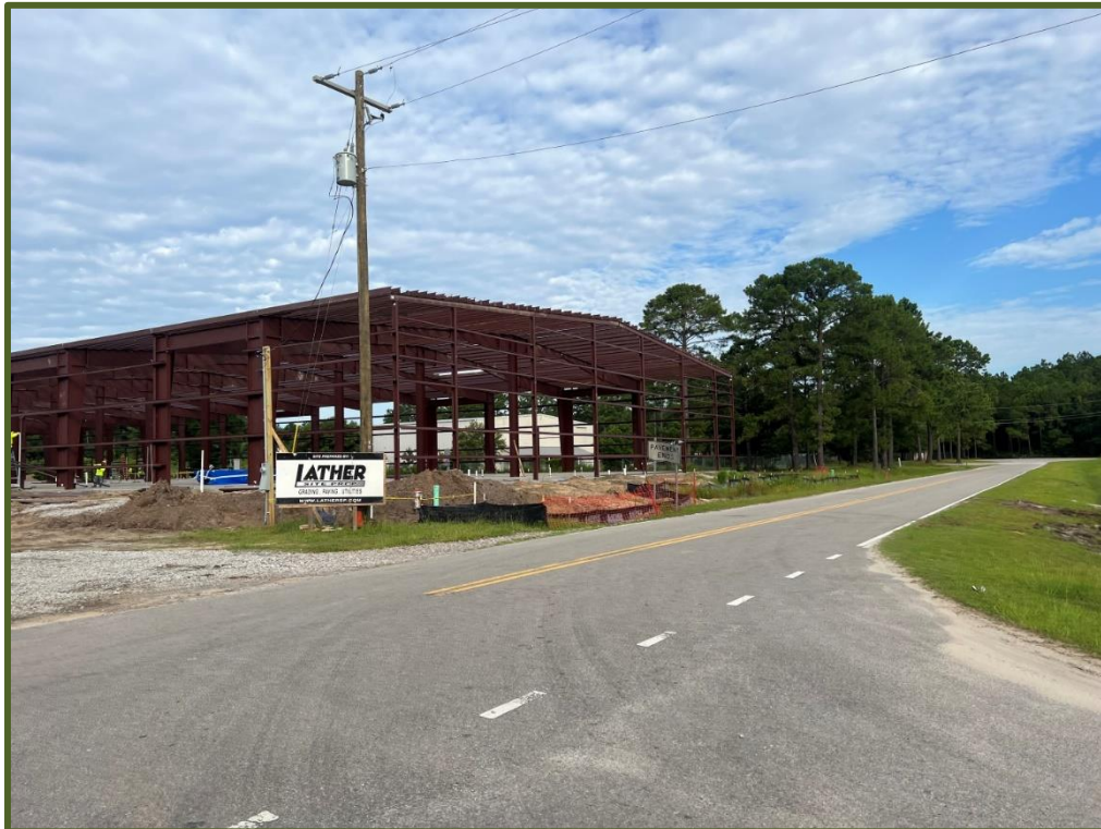
New Construction Underway in Development
