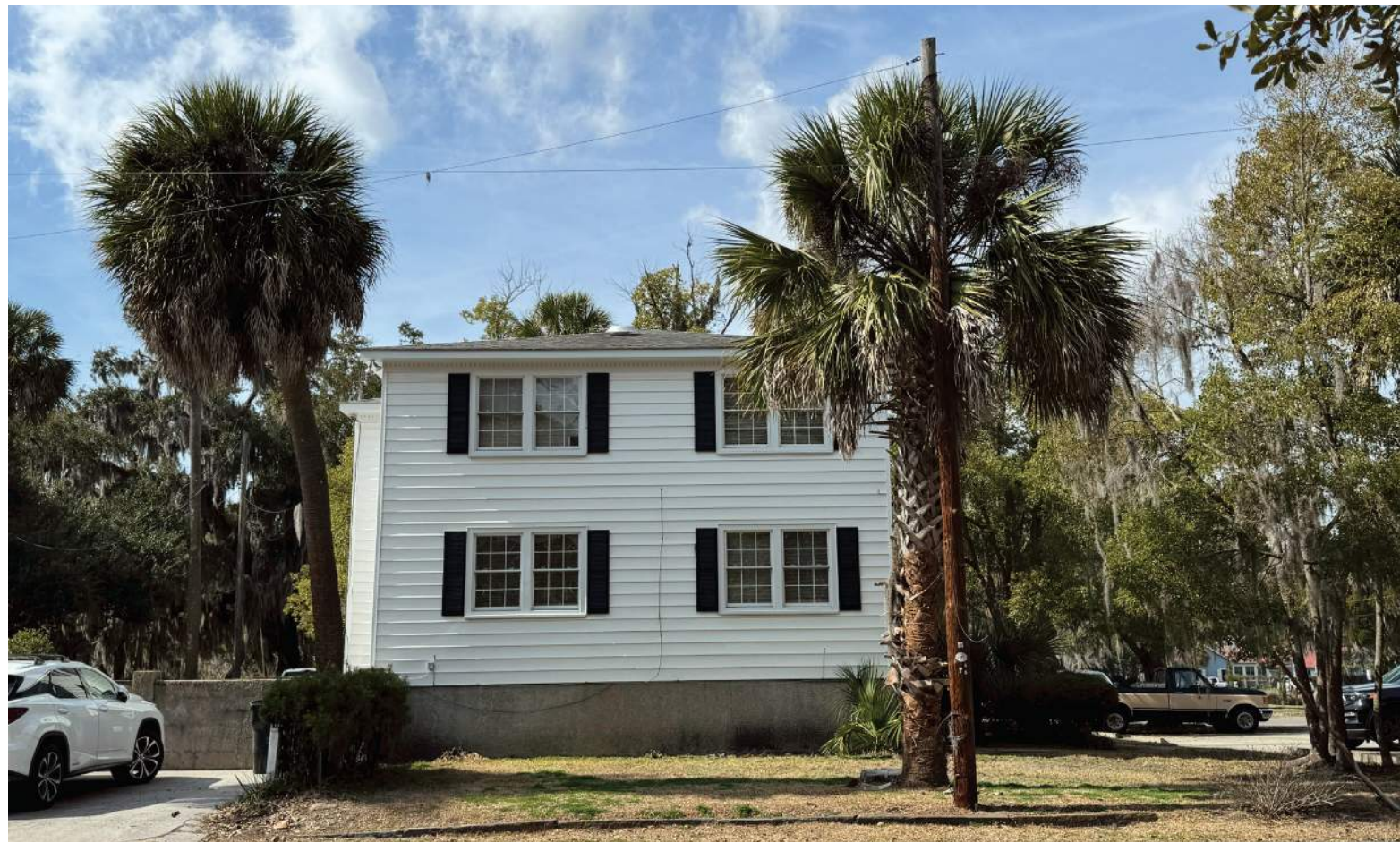
ACCESSORY STRUCTURE ACROSS MONSON, WEST OF 1411 NORTH STREET
