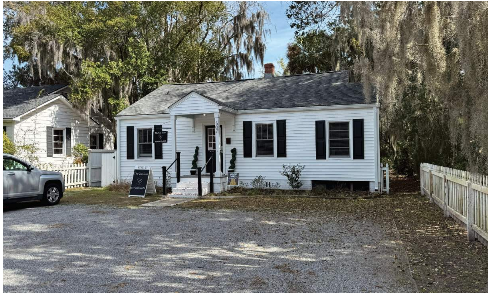
ADJACENT OFFICE BUILDING TO NORTH OF 1411 NORTH STREET
