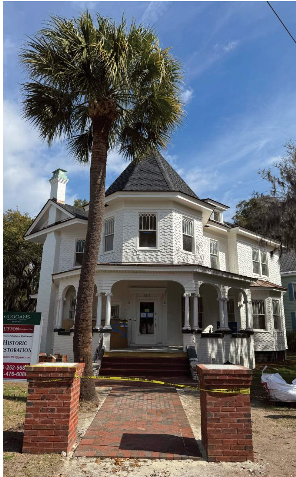
1411 NORTH STREET - FRONT OF HOUSE SHOWING PIERS
