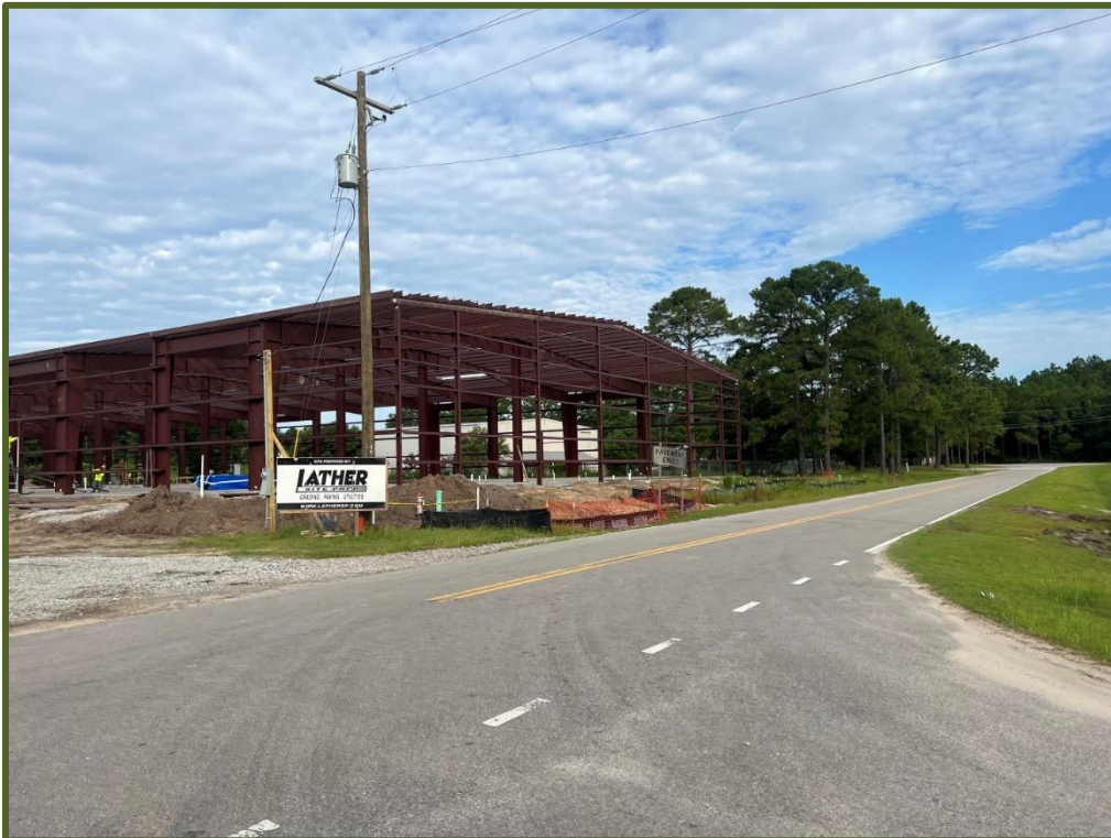
New Construction Underway in Development
