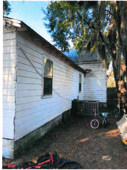
EAST SIDE - FIBER CEMENT SIDING
