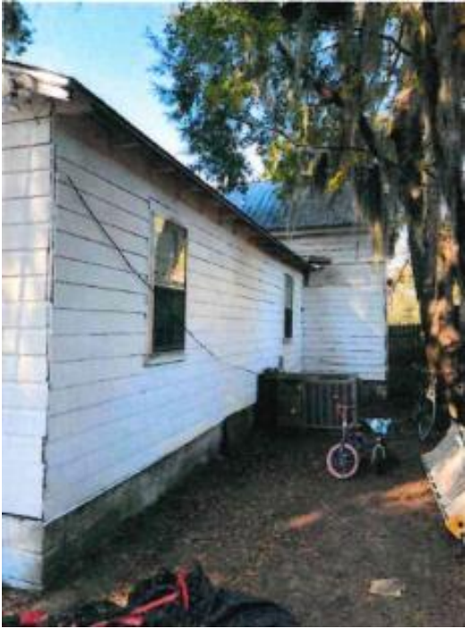
East side: Fiber cement siding (existing)
