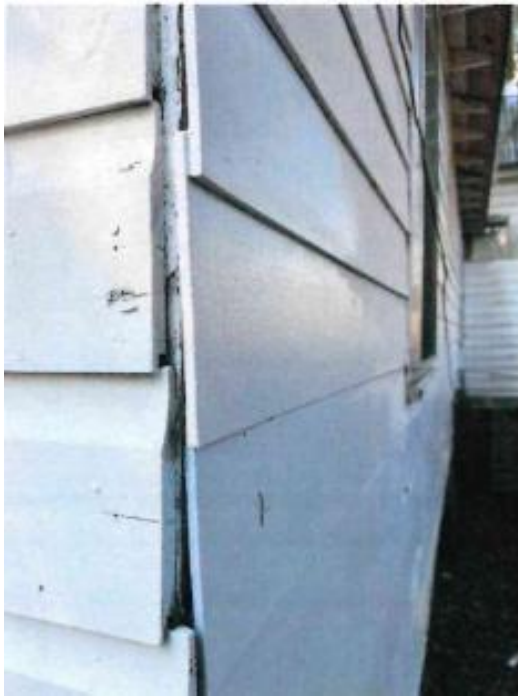
Fiber cement siding (close-up)
