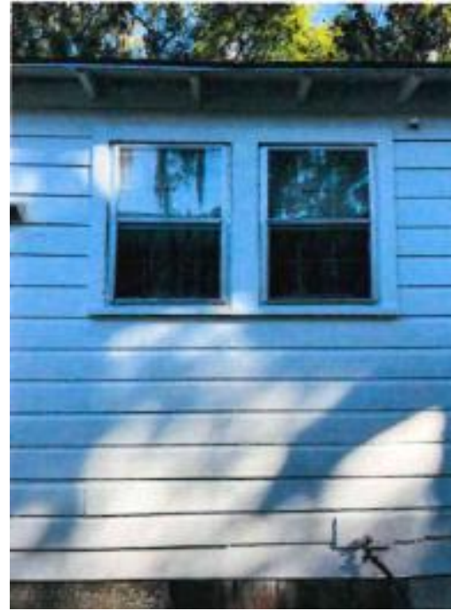
Existing kitchen windows (close-up)
