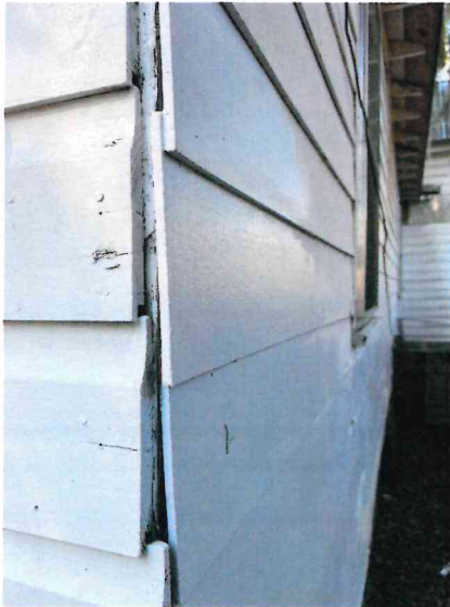
FIBER CEMENT SIDING CLOSE-UP
